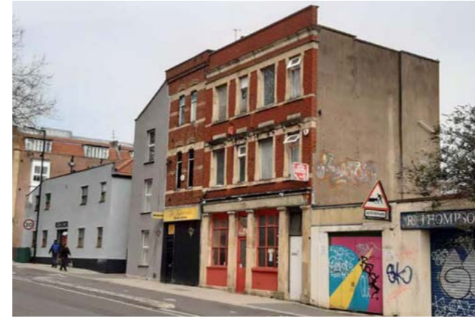
Existing Whitehouse Street frontages
