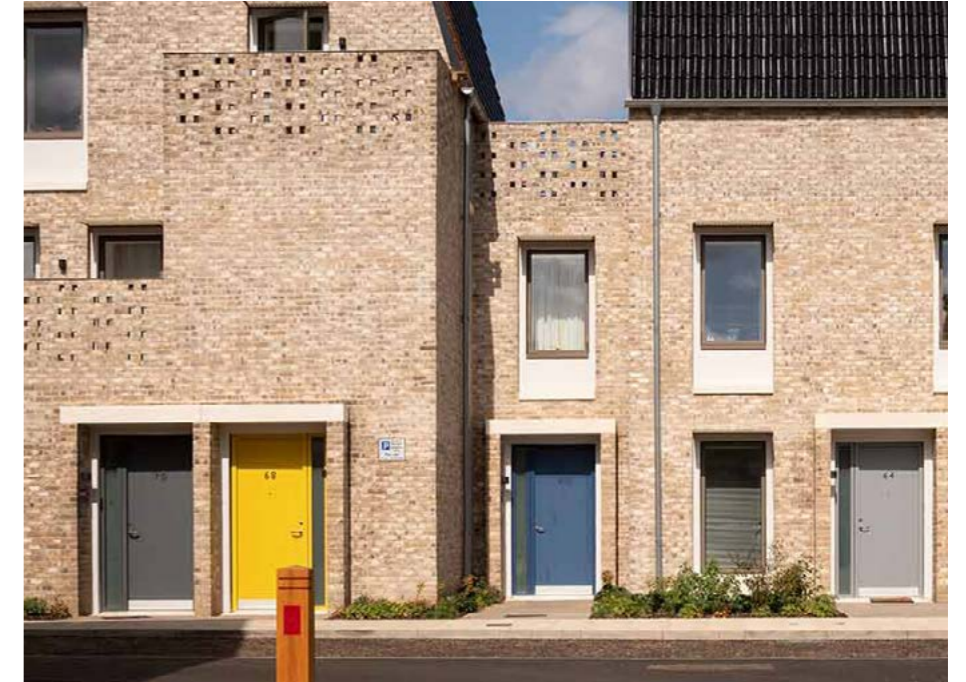
Goldsmith Street, Norwich. The detailing of ground floor entrances adds a texture and variety at eye level.
